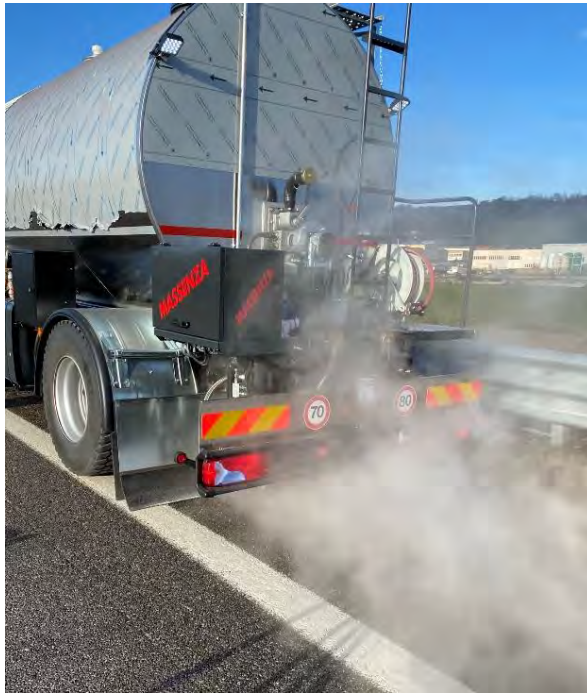
Figure 7 - Phyto-based salt brine application on highway porous asphalt pavement
